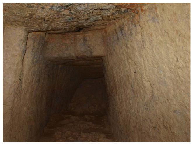
Fig 11 Roman mine gallery with trapezoidal cross-section in the Cârnic massif.
