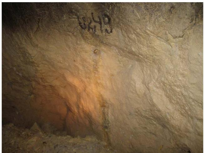
Fig 18 Shothole for explosive charge in the wall of an early modern mine gallery in the Cârnic massif.
