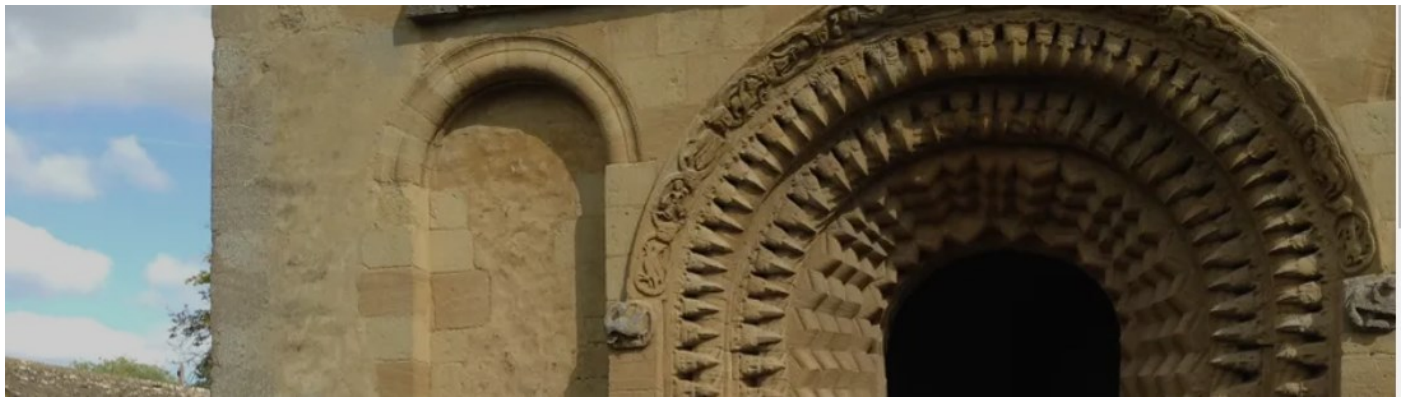
The West porch of the Norman church St Mary, Iffley
